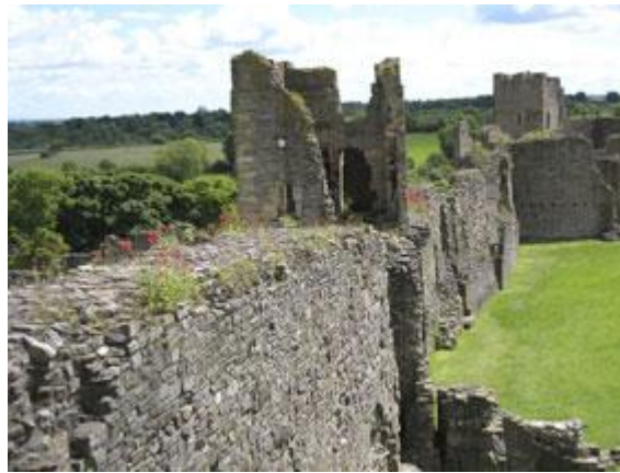
A ruinous part with a pretty bit of wall
