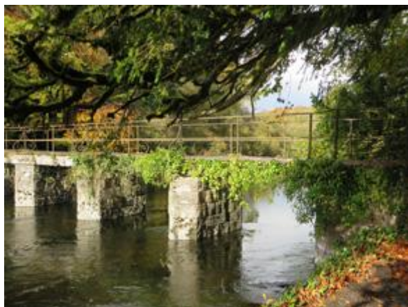
Bridge over the River Cong
