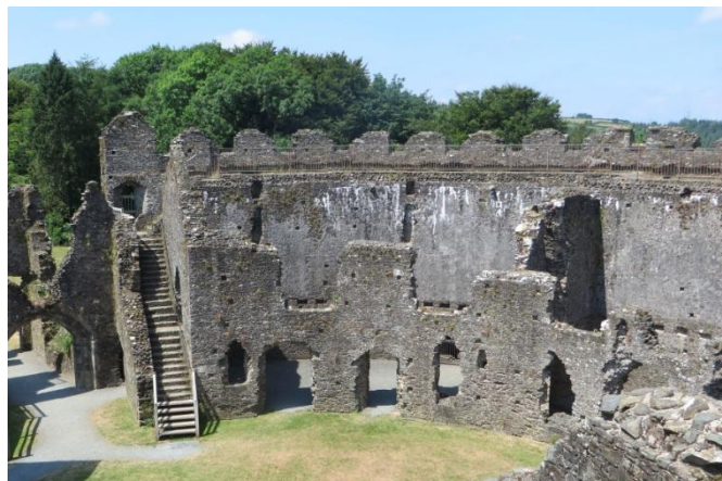
Steps leading up to the wall-walk
