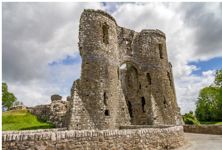
Side view of the double-drummed gatehouse (photo by Alan Santillo)
