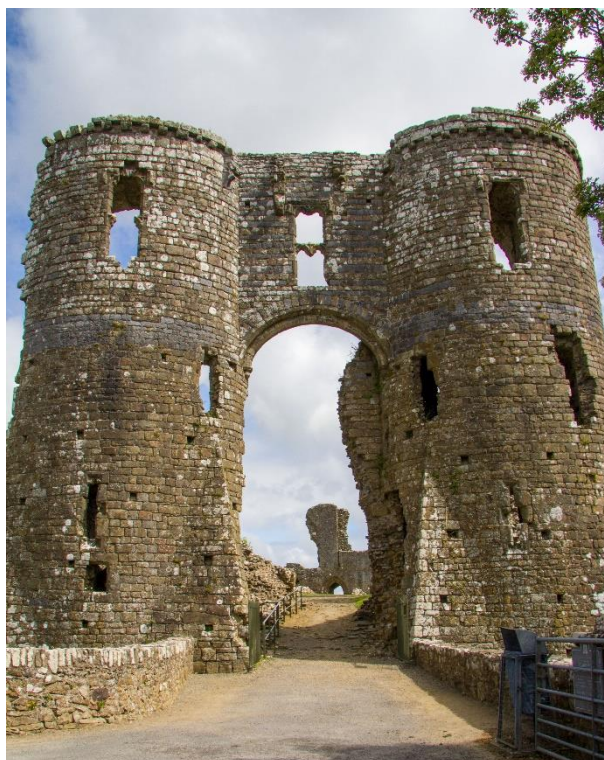
The gatehouse (photo by Alan Santillo)
