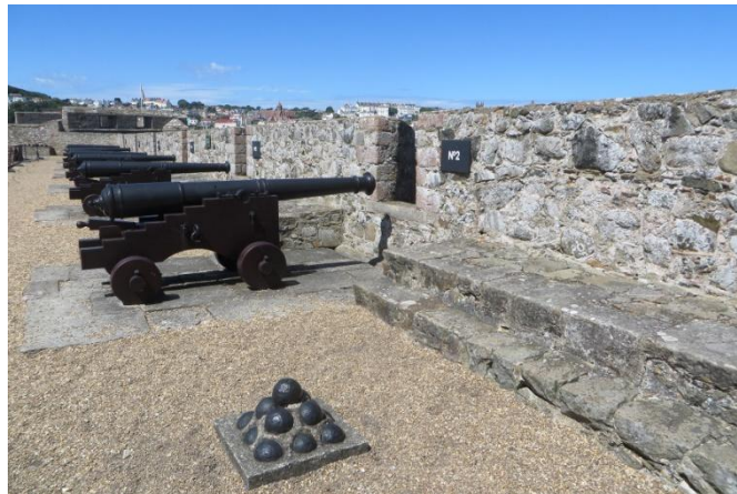
Cannons, balls and massive walls
