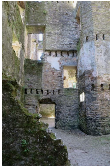
Within the empty rooms
