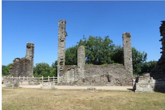
Remains of the north wing and loggia
