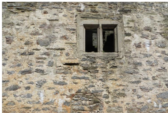
A 'Seymour wall' - and window, presumably!
