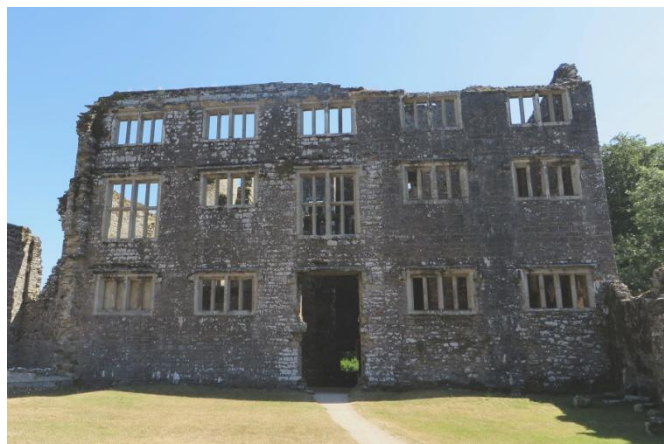
Remains of the Elizabethan building
